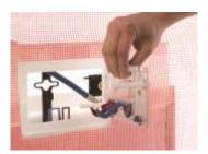
The grey locking nuts are turned anti-clockwise and the inspection cover can then be removed.
