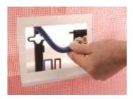
Undo the hose connected to the inlet valve and remove grey outlet valve hold down devise.
